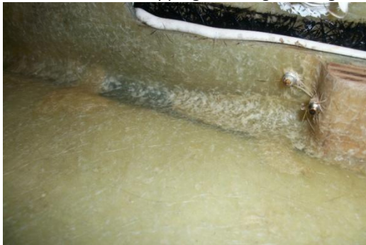
Fig 4 Underside of forward hull and deck
