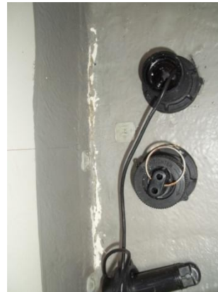
Delaminated bulkhead
