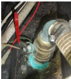
Toilet skin fitting and valve for reference.
