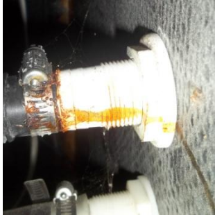
Forward bilge pump outlet leaking.
