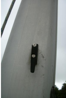
Fig 20 Mast cleat broken
