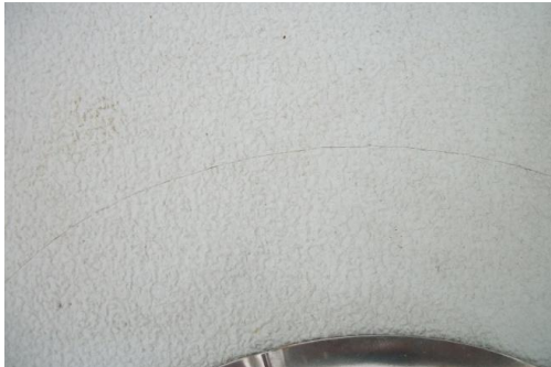
Fig 6 Deck “cut” around vent
