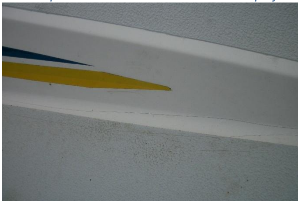
Fig 7 Stress crack starboard side deck
