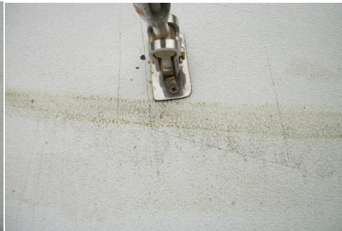
Fig 6 Deck “cut” around chainplate.
