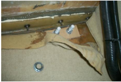
Fig 21 Beaching posts internal fitting
