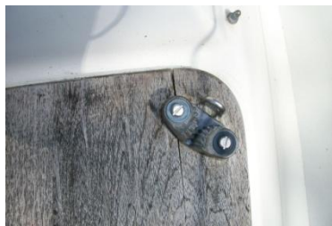
Fig 9 Teak ply coaming detail
