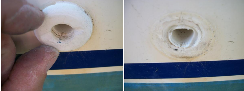
Fig 8 – 9 gas locker drain before and after testing
