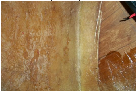
Fig 5 Well bonded floor panels
